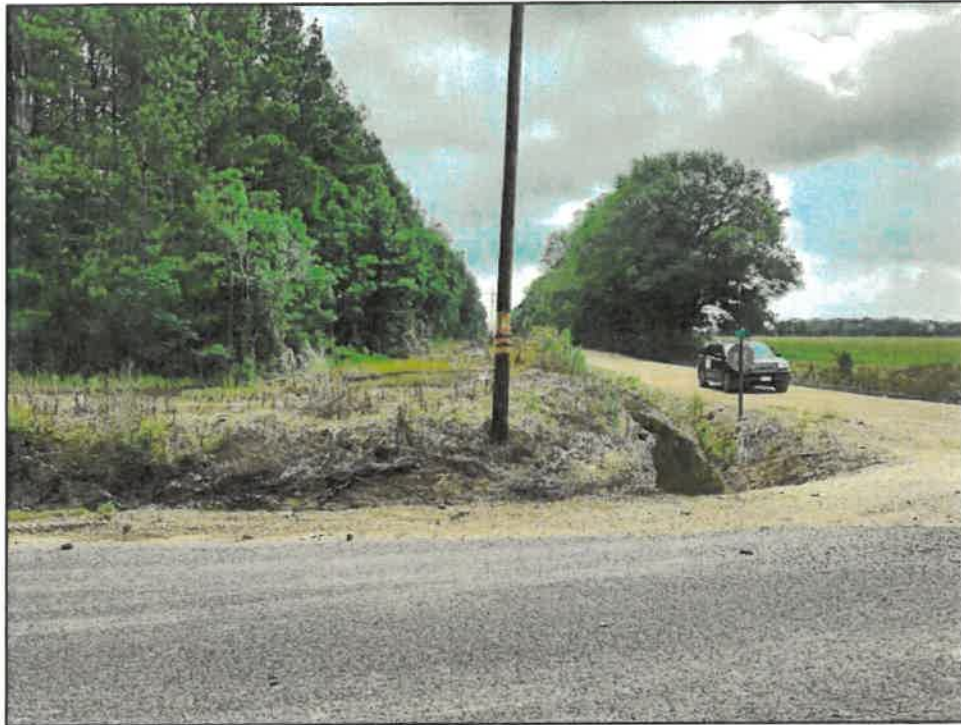
Figure 5.10. View of Bel Oil road crossing through the project area, facing east.
