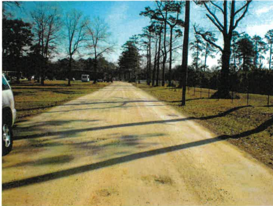
Figure 3.2 West end of Maintenance Road Project Area (looking east)
