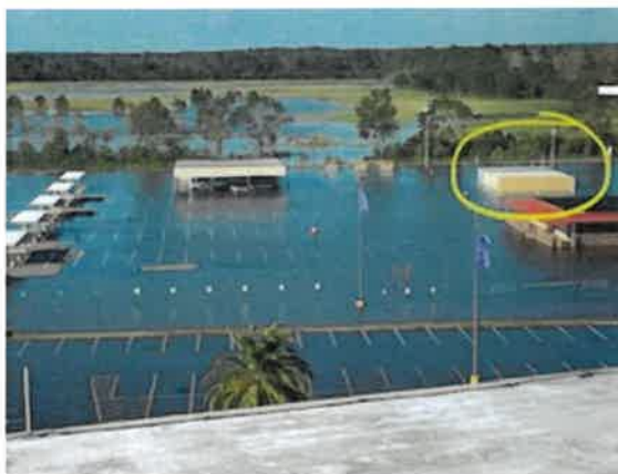
Figure 9-23 Floodwaters Infiltrating Various Tribal Facilities
